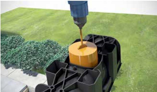
Produce connection openings.
