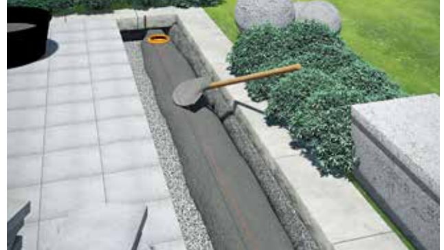
Fill with concrete and compress to foundation.
